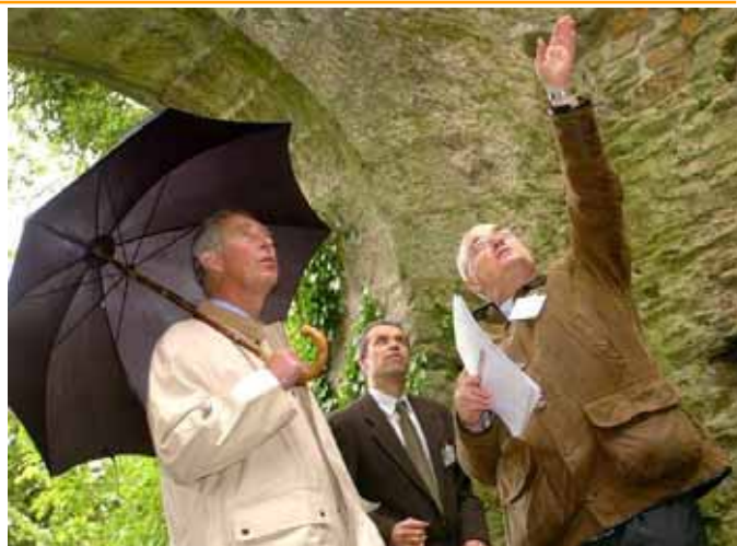
Prior to the presentation, His Royal Highness was shown a consolidated engine house at Holmbush Mine in the company of Nicholas Johnson, Historic Environment Service Manager (right) and Chris Hariades, Environmental Programmes Project Development Officer (centre)
