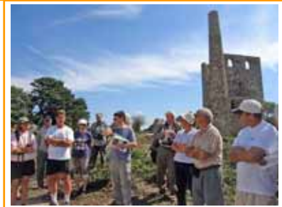
Above: Ainsley introducing the site and explaining the recent building consolidation work. The 70 inch cylinder pumping engine house can be seen to the rear. Image Sharron Schwartz 2007
